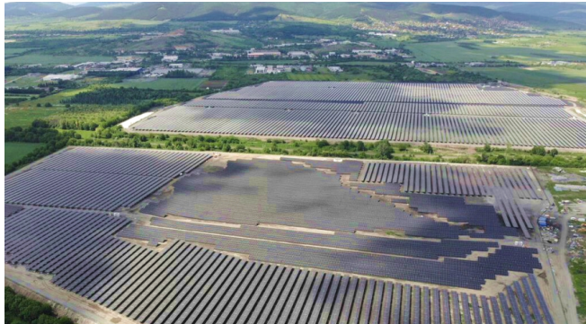
Bulgaria C Solar Project 109MW
