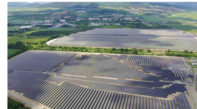
Bulgaria C Solar Project 109MW
